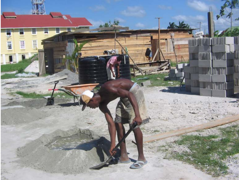
Picture 2: Workmen on site preparing to lay foundation for recreational centre
